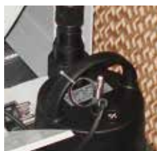
GRUNDFOS WATER PUMP WITH FLOW REGULATION AND CONTINUOUS DRAINAGE SYSTEM TO AVOID MINERAL SALT CONCENTRATION.
