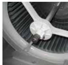
ROULEMENT AVEC TRAITEMENT ANTICORROSIF CORROTEC + COUVERCLE DE PROTECTION.
