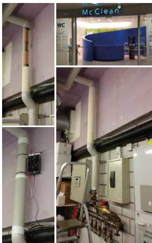
Vulcan anti-scale system in the hygiene center of the station in Basel.
