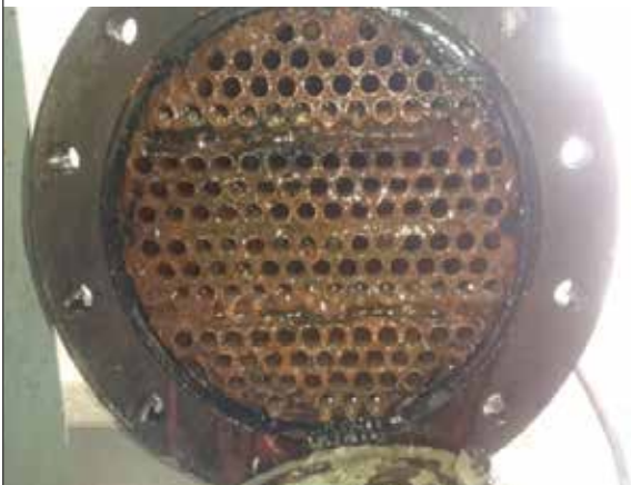
Heat exchanger before Vulcan installation
