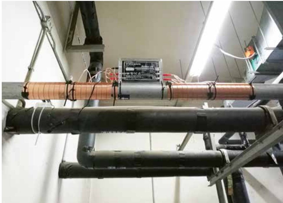
Vulcan S25 installed on the main water pipe of the cooling tower.
