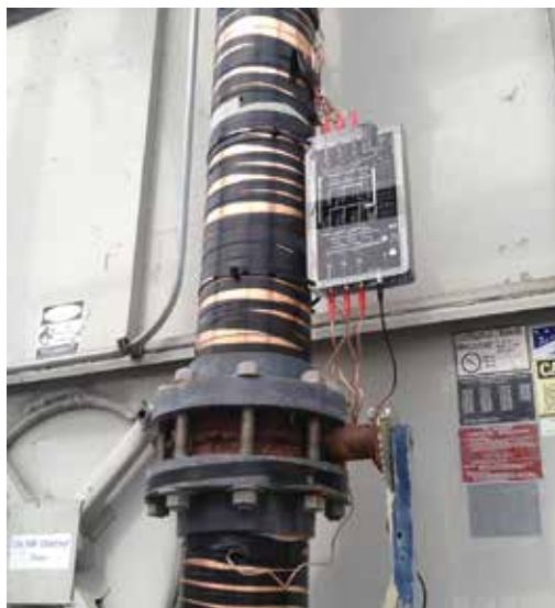
Vulcan S100 installed on cooling towers
