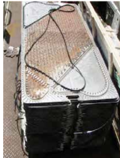
After Vulcan was installed for 9 months: the plate heat exchanger was taken apart for cleaning.
