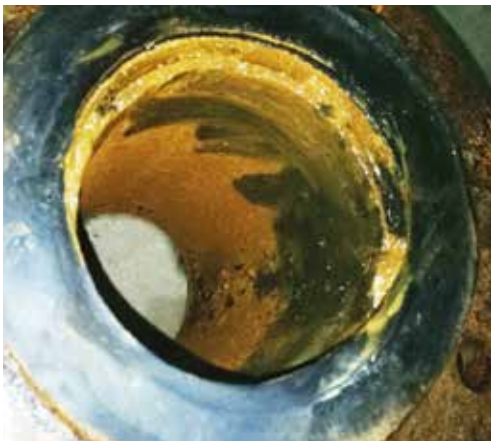
Scale can be easily wiped off, and the pipe shows the smooth wall
