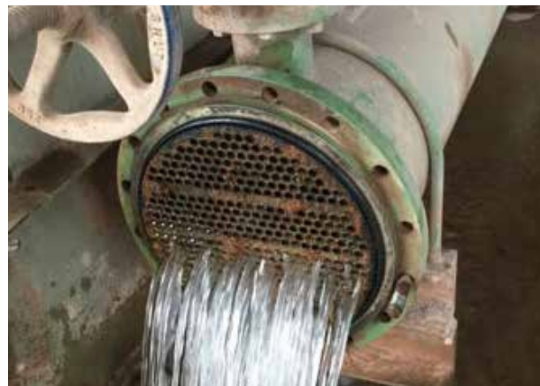
Heat exchanger after 2 months Vulcan installation
