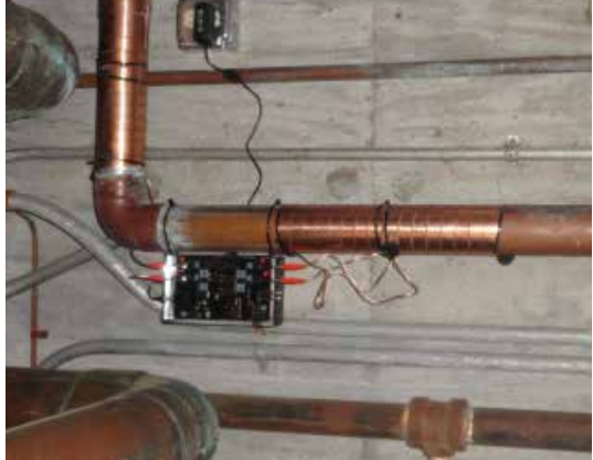
Vulcan unit installed on water main
