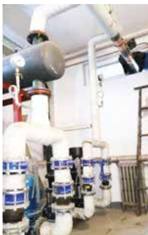
Vulcan S25 for solving the shower head scaling problem.
